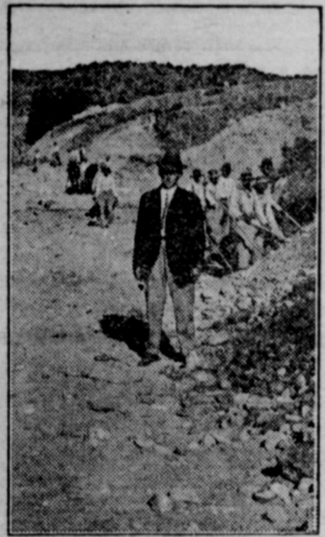
Convicts Building Good Road.
