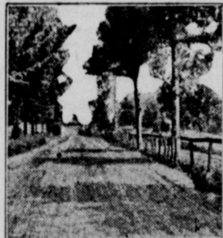
Macadam Road Treated With Asphalt Binder.
