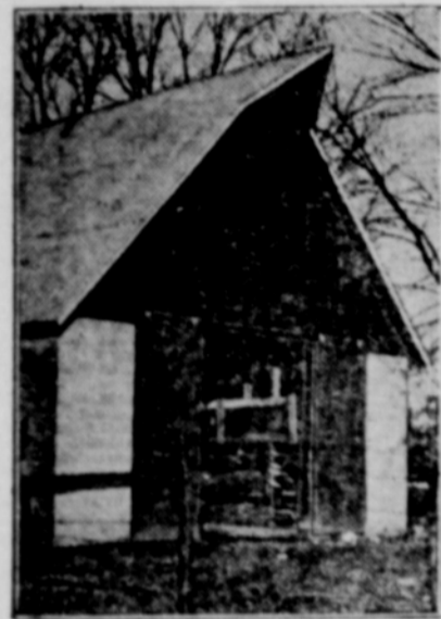
A Permanent Concrete Crib.
