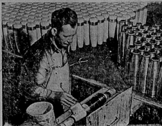
Shaving a 7.2 inch howitzer shell on a giant lathe. The Dominion's ammunition factories make 18 types of shells in 14 different calibres. They employ 50,000.
