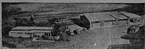
The photograph above shows the new quarter-million-dollar plant of the Wynn Oil Company of Azusa, California, completed early last year. This factory is considered one of the most modern processing plants in the entire United States. Designed by the Austin Company of Cleveland, Ohio, it features fully automatic push-button control in its mixing and blending processes.
