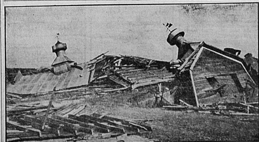
IN THE WAKE OF A TWISTER—A death-dealing tornado struck Rhineland, Wis., killing two and injuring 50. In the wake of the violent wind storm, which caused untold damage, lay shambled barns and homes grim reminders of nature's fury.
