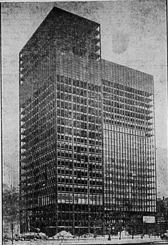
PEOPLE IN GLASS HOUSES —The entire outside of this 28-story apartment building in Chicago is made of steel and glass. When completed, the structure on Chicago's Lake Shore Drive will have more glass than the Merchandise Mart, which is the world's largest building. Two garages will be located in the basement and sub-basement of the "Glass House."
