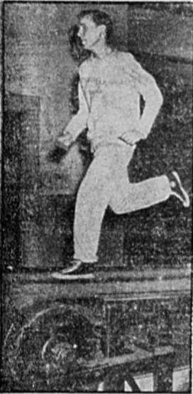
GOING NOWHERE FAST— Students at Cincinnati's Central Vocational High School built a treadmill to help their track team beat the rainy spring weather. The belt, which simulates conditions on an indoor track, can be set, at speeds to satisfy both sprinters and distance men.
