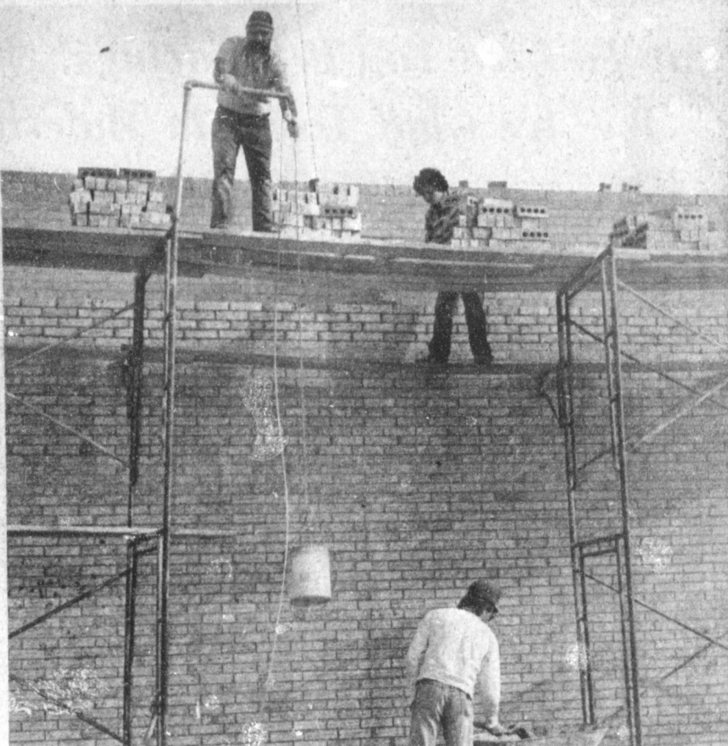
WORK NEARS COMPLETION...The relaying of brick on the south side of Muleshoe Super Market which was damaged by fire earlier this year is almost completed. The last few pretty days have enabled the workmen to get in some good time on the job. Tony Luna is the contractor on the job.
