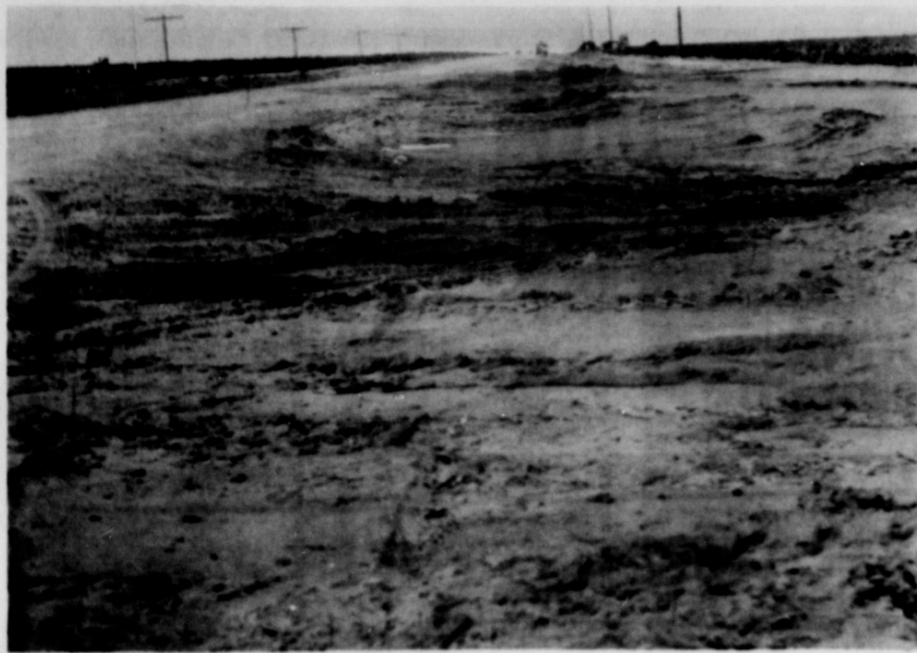
RAIN WASHED MUD COVERS HIGHWAY 70 SUNDAY after the torrential downpour Saturday night. This view was taken one and one half miles west of Earth. The highway was closed at 3 a. m. to 10 a. m. Sunday, due to the water and mud.
