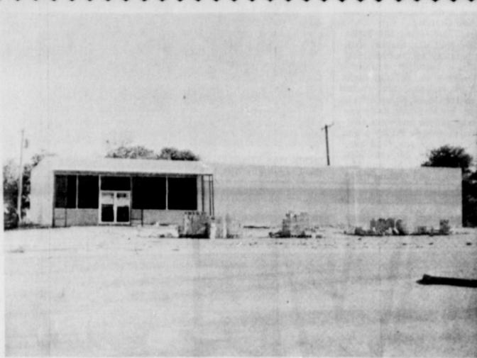
**PIGGLY WIGGLY BUILDING NEARS COMPLETION...** as shown in the picture. The spacious \$30,000, building will house the present supermarket, which is located on the corner of Main and 1st Street. The 100'x60' building is of tile structure and the exterior has been finished in ivory. The building will feature all new metal display fixtures, when completed.
