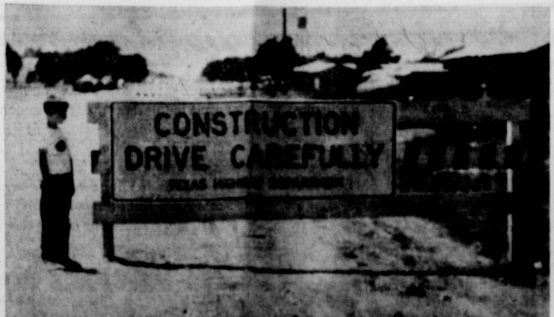
LOOKS LIKE THEY ARE GETTING DOWN TO EARTH, by the sign that was erected here Tuesday. The heavy machinery is arriving and things are shaping up to begin construction on the four-lane drive through the City of Earth. One and one-eighths mile through town will be widened. Looking at the sign, hopeful that they will begin soon is 9 year-old Phil Middleton.
