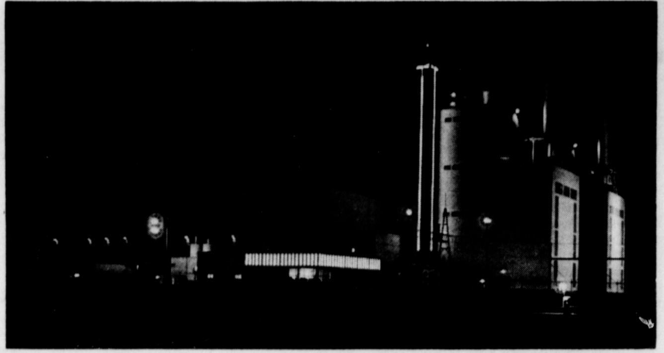
Clifford B. Jones Station is Southwestern Public Service Company's largest generating plant. It is located southeast of Lubbock on Farm Road 3020, just west of the Buffalo Springs Lake
