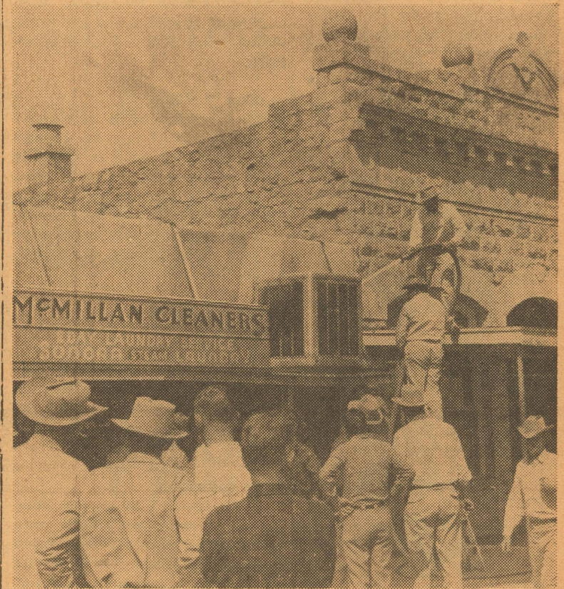
PROMPT ACTION by Eldorado firemen prevented the spread of the fire which gutted McMillan Cleaners last Friday.
